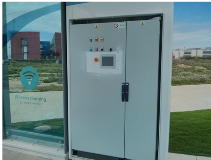
Figure 25 Power electronic cabinet Installed including the HMI
