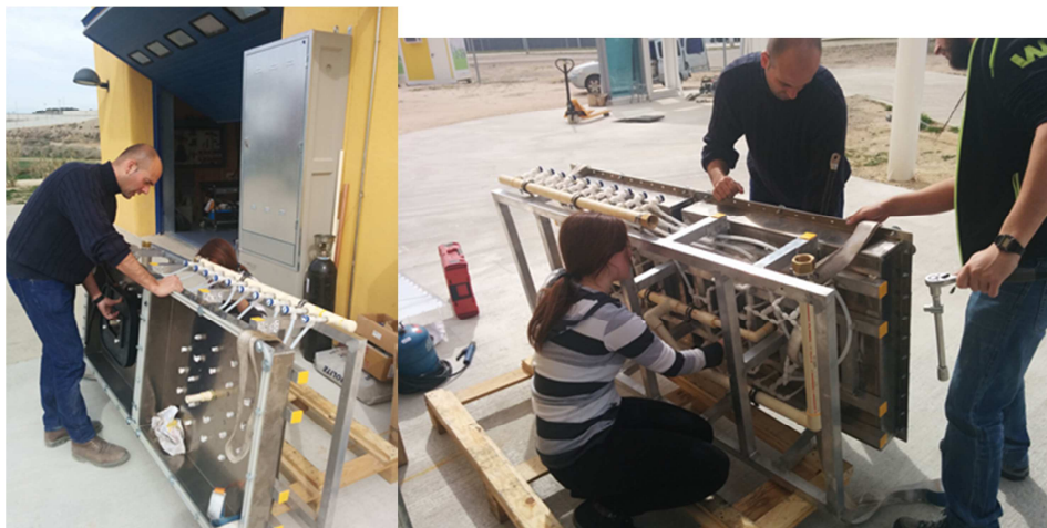
Figure 19 EMI shielding and cooling pipelines
