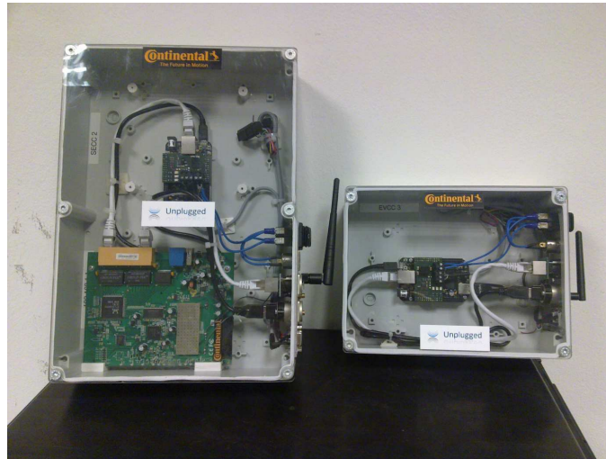
Figure 61 - Prototype of wireless communication system for UNPLUGGED (SECC on left side)
