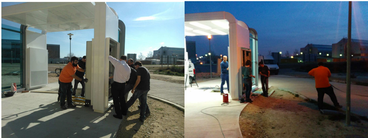
Figure 24 Installing Power electronics in the charging station
