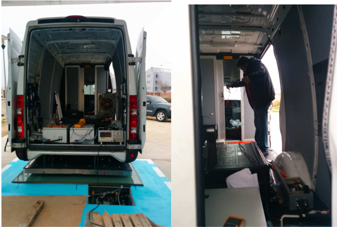
But finally, the work was done and the rain allowed taking nice photos of the charging station
