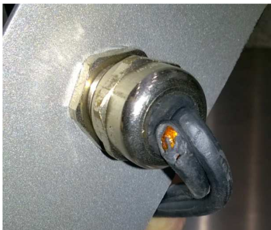
Figure 55: Damaged cable due to unfavourable mounting construction
