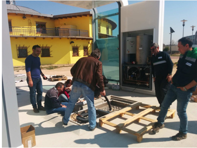
Figure 18 Installing the oil cooling system
