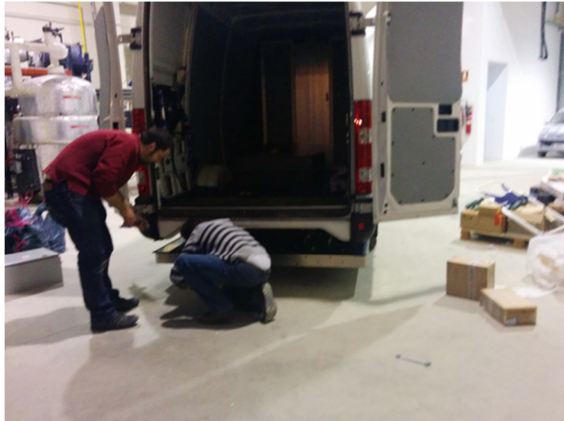
Figure 13 Installing secondary coils and EMI shielding
