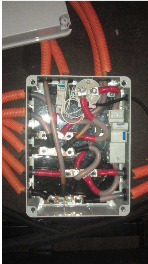
Figure 11: HV Distribution Box
