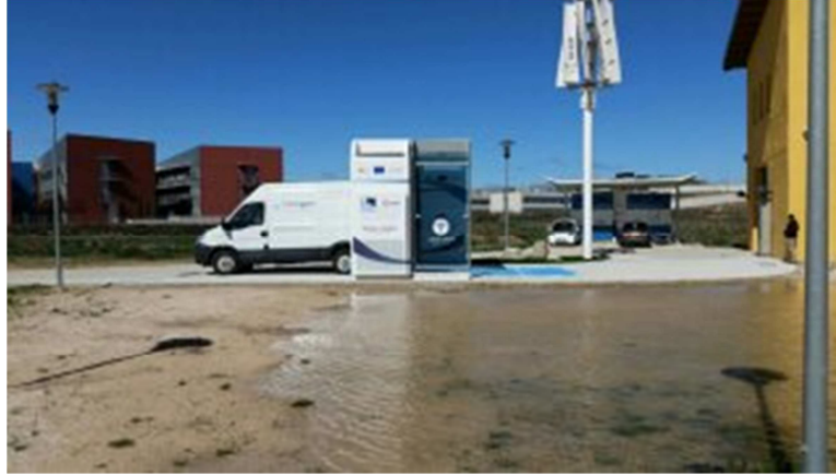
Figure 36 Charging station at CIRCE facilities
